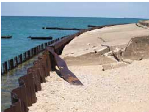
Recent photos show severe damage to Point Betsie Lighthouse's essential Shoreline Protection System (SPS). Photo Credit: Walk Softly Photos.
