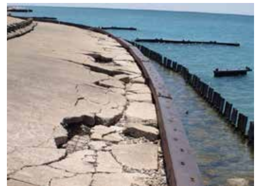
Recent photos show severe damage to Point Betsie Lighthouse's essential Shoreline Protection System (SPS). Photo Credit: Walk Softly Photos.
